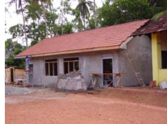
Re-building school library
